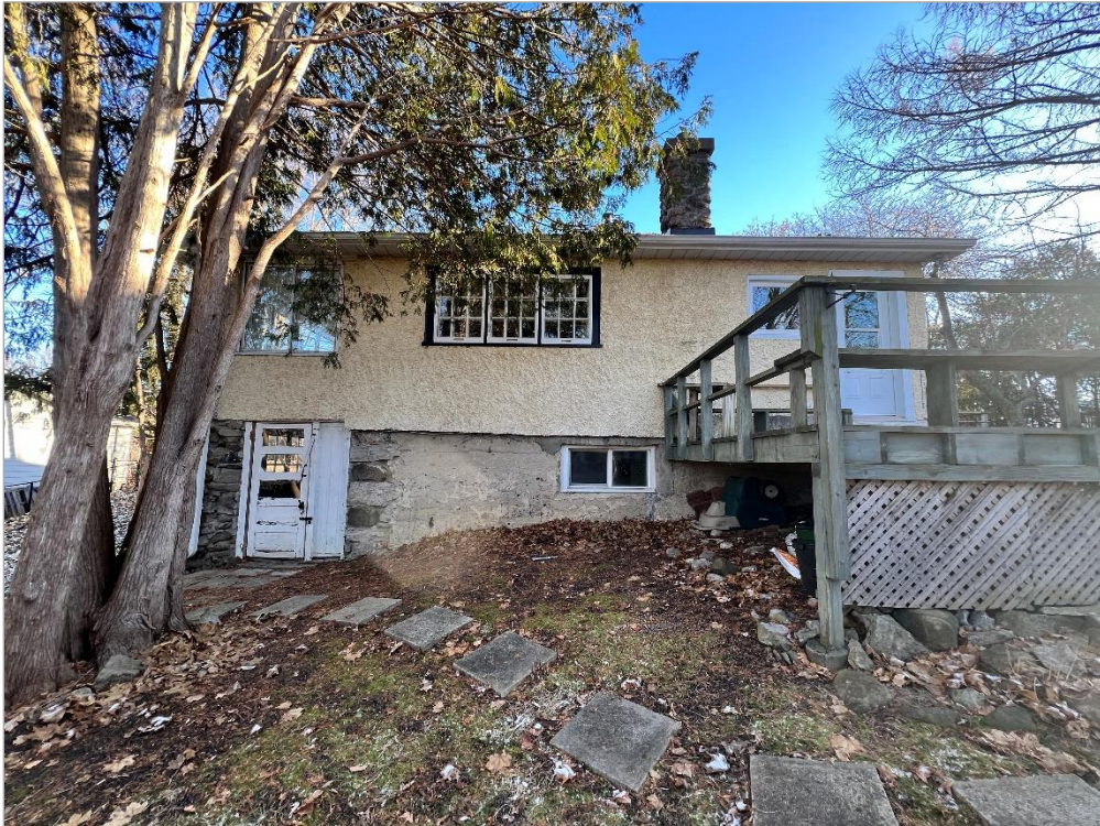
Rear view of the building
